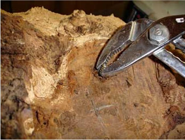
17. Next use a pair of pliers to remove the broken screw.
