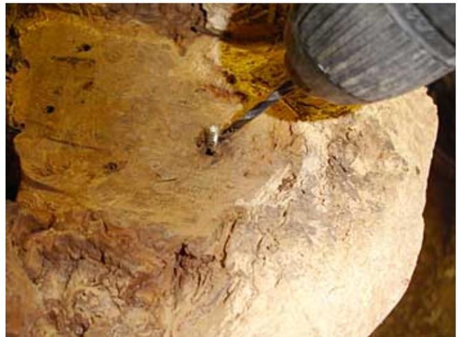
16. Start with a 3mm or 4mm drill bit and drill holes right next to the screw. Use a drill bit suitable for metal. Try and drill as close to the screw and as deep as the screw. Drill as many holes as possible and then angle the drill as shown above to break through the adjoining holes.
